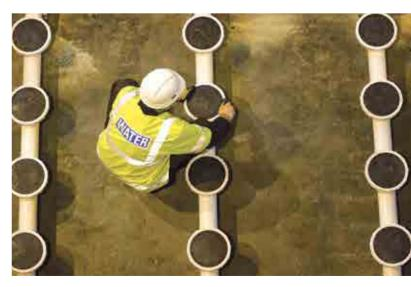
Upgrading of air delivering system to save energy
